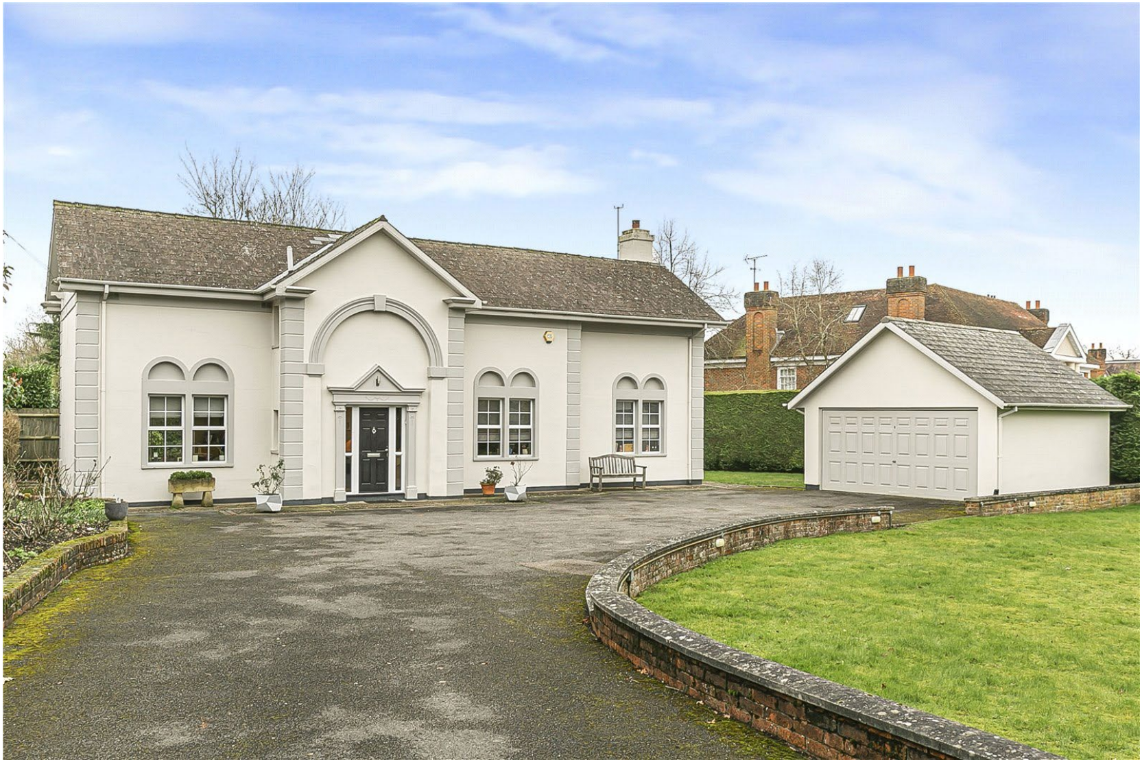
THE COACH HOUSE, 46a Totteridge Common, Totteridge, N20 8ND
